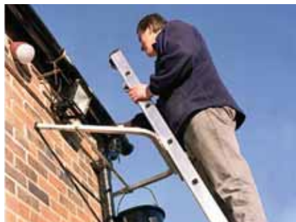
Fig 41. Ladder stand-off device in use
